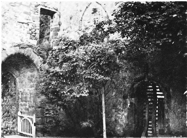
MILLOM CASTLE : Courtyard with entrance to the great chamber.
