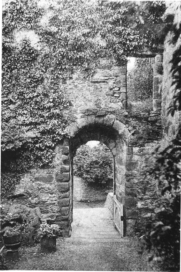
MILLOM CASTLE : Courtyard with entrance and door to chapel. Phot. by Mr. W. L. Fletcher. TO FACE P. 187.
