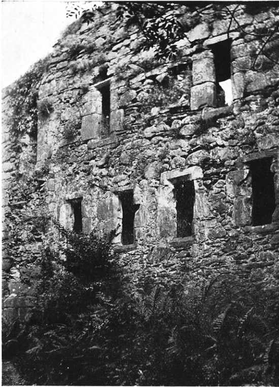
MILLOM CASTLE : exterior of the kitchen.
