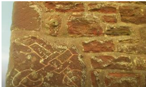
Part of a 10 th Century Cross embedded in Church Wall
